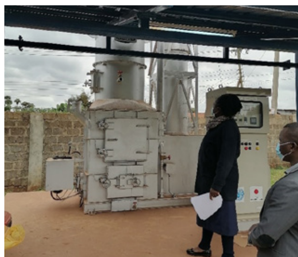
Figure 16: Officer-In-Charge of Mutuini Hospital explains how the new incinerator works. This was donated through UNIDO/JICA sponsorship in Kenya
