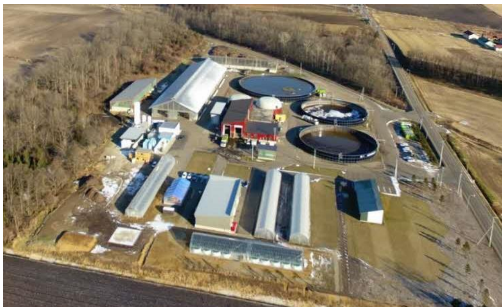
Naka-Shikaoi Biogas Plant
