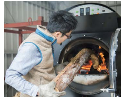
Firewood boiler at hot springs facility
