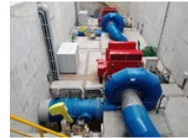
Hydro Power Plant, Chodai Co., Ltd., Philippines
