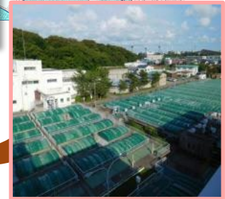
Akita City WWTP (Only for rainwater treatment from 2020)
