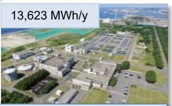
Akita Rinkai WWTP
