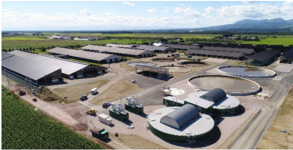
Biogas power generation facilities
