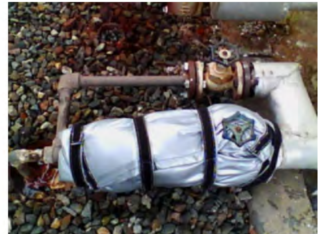
Example of insulation around steam trap
