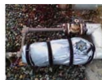
Example of insulation around steam trap
