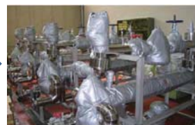
Example of insulation around steam trap
