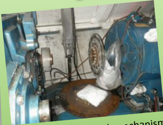
Remove coupling break mechanism
