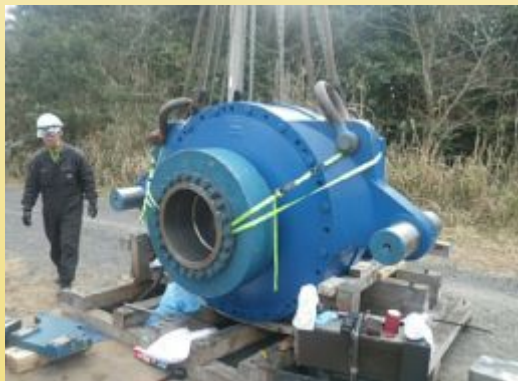
Hoist new gear box
