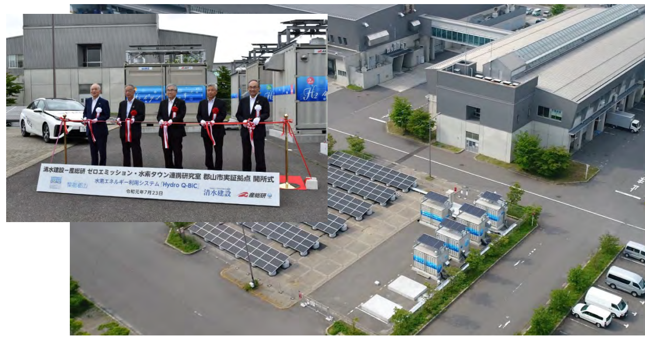
Hydrogen energy system for buildings at Koriyama City General Wholesale Market
