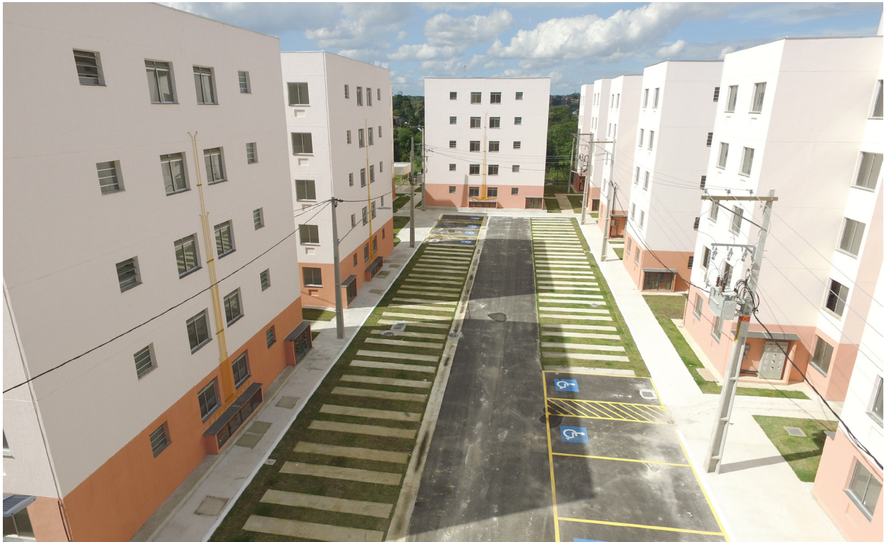
New housing units built.
