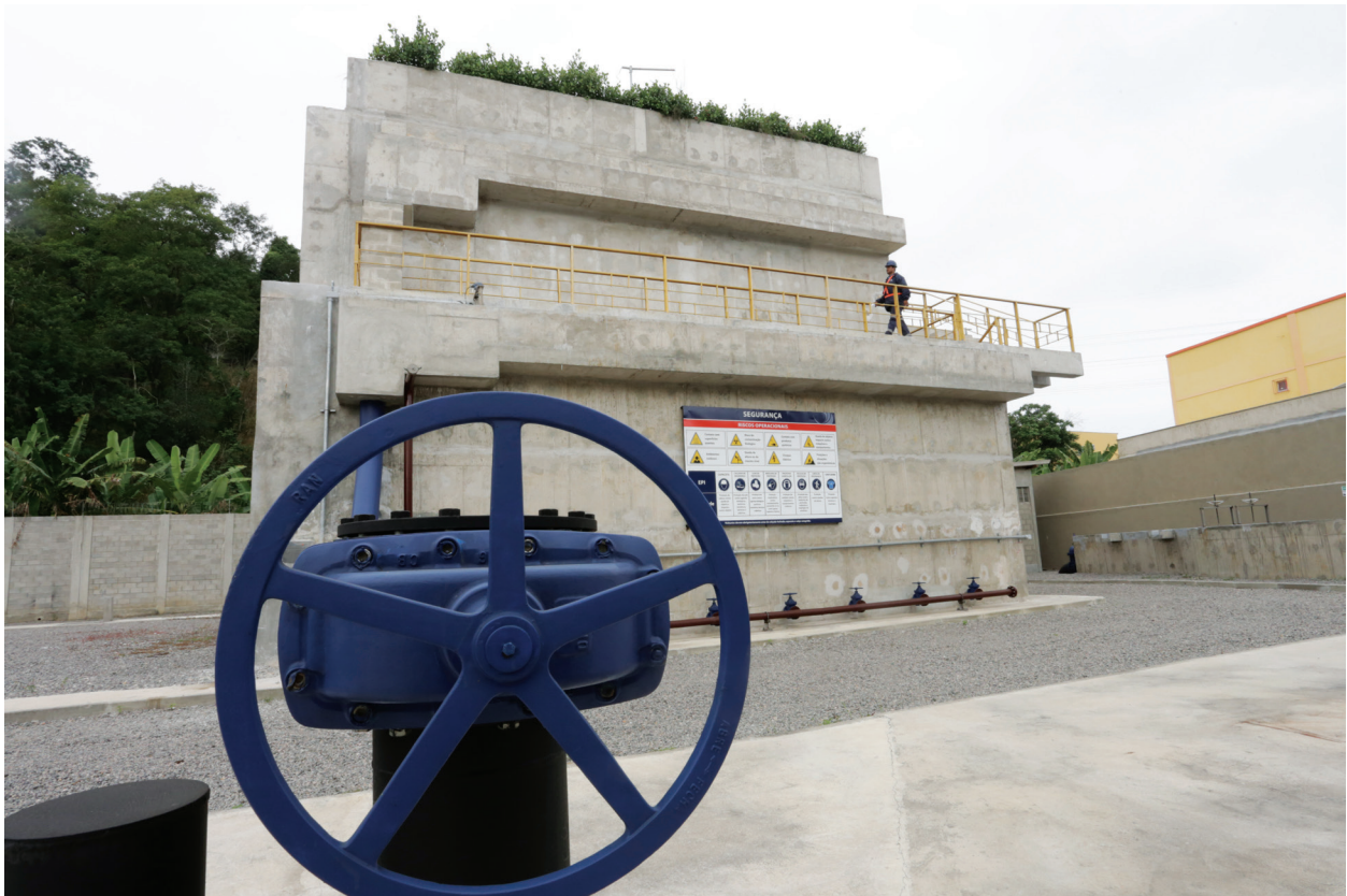
Sewage Treatment Plant (ETE) Maria Paula.
