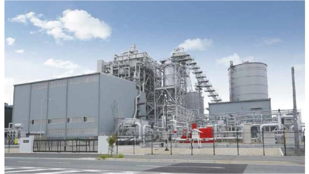
Hibiki Coal and Biomass Power Station (Hibikinada Energy Park LLC.) Generation capacity : 112,000kW
