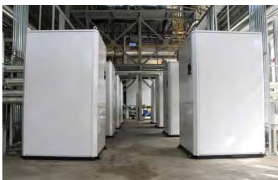
Heat recovery heat pumps
