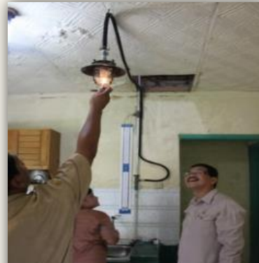
Methane capture from septic tank
