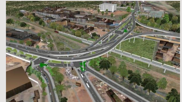
[Loans] Kampala Flyover Construction and Road Upgrading Project (Uganda)
