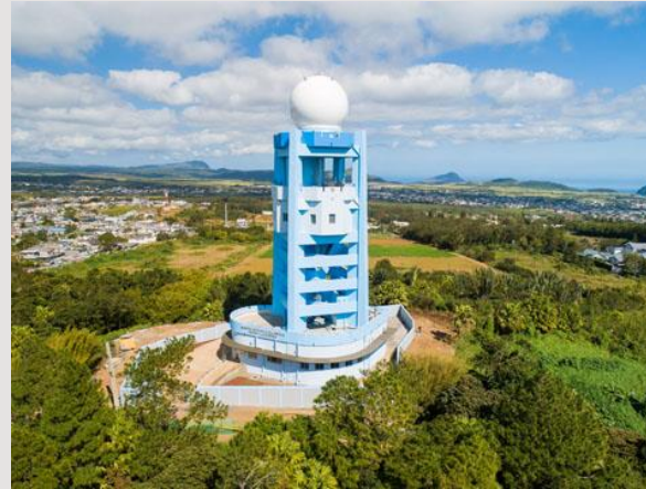
Improvement of meteorological radar system (Mauritius)
