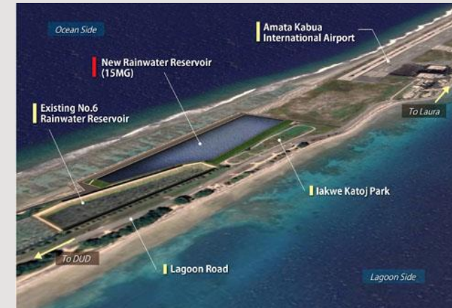
[Grant] The Project for the Improvement of Water Reservoir at Majuro Atoll (Marshall Islands)
