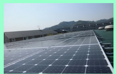
Solar power generation
