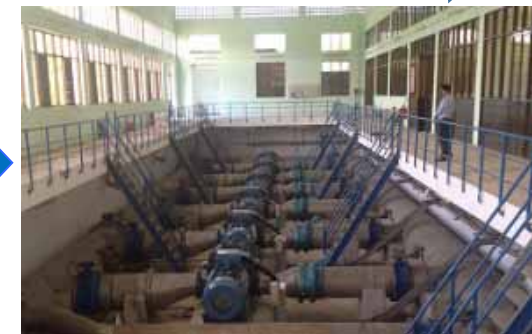
Replacement of pumps at water purification facility (Joint Credit Mechanism-supported project)
