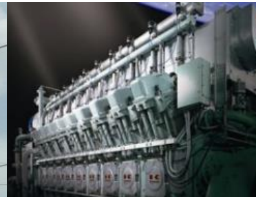
Co-generation system at factory, Toyota, Nippon Steel & Sumikin Engineering, Indonesia, Thai
