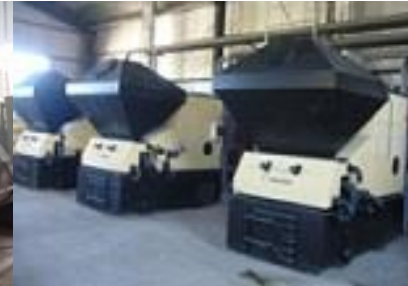
High-efficiency Heat only Boilers, Suuri-Keikaku, Mongolia
