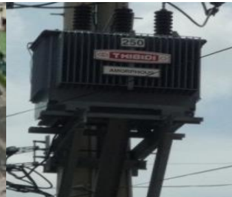
Amorphous transformers in power distribution, Hitachi Materials, Vietnam
