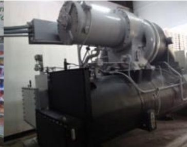
High efficiency air-conditioning and process cooling, Ebara refrigeration equipment & systems, Indonesia
