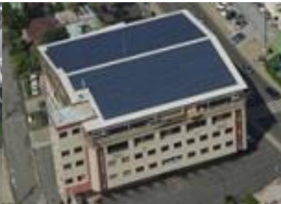
Installing solar PV system, PCKK, Palau Maldives
