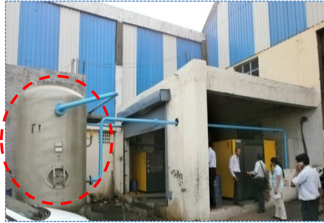
Installation of new receiver and new air compressors (not inverter type)
