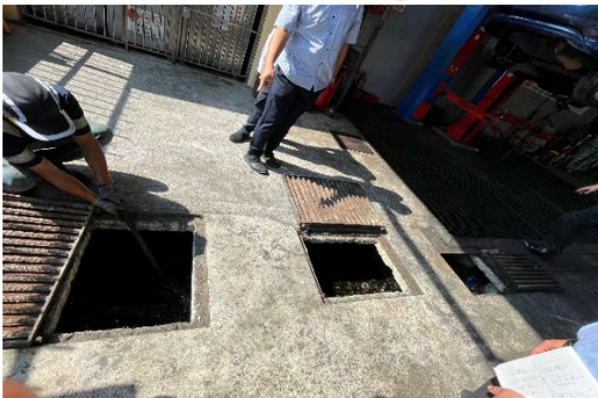
Leaked Liquid Filtration (3-step system, left to right)
