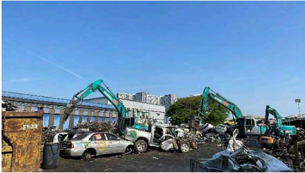
Final Dismantling Area
