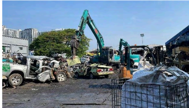
Dismantling Using Nibbler
