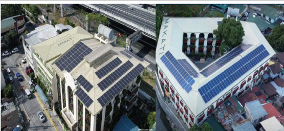
Solar Panels in Schools
