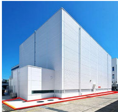
Cast-in-place concrete (within red frame)
