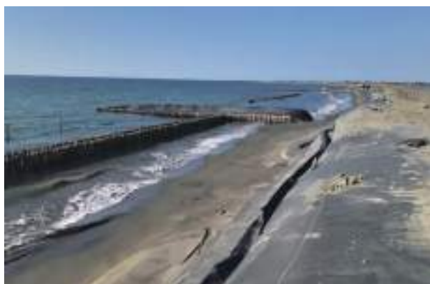
△ Bamboo Stakes and Sand-Filled Tubes Installed at Qingshan Port Sandbar to Dampen Wave Impact
