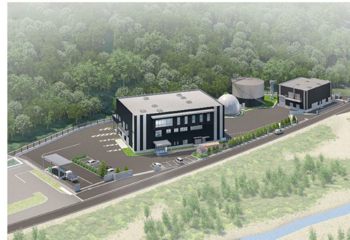
Image of food waste recycling facility (expected to be operational in 2024).
