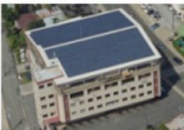
Installing solar PV system
