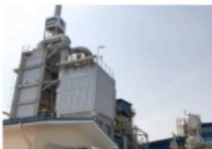
Waste to Energy Plant
