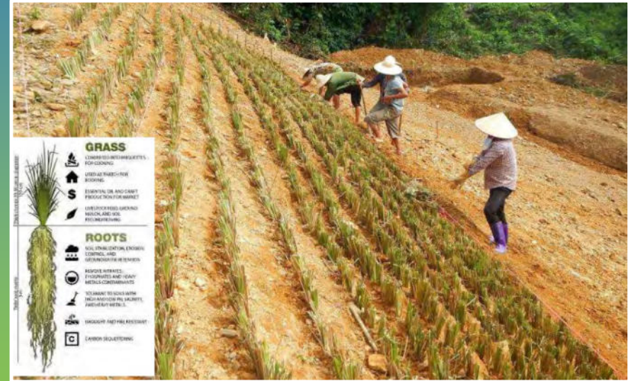
Fill slope: Vetiver grass lines
