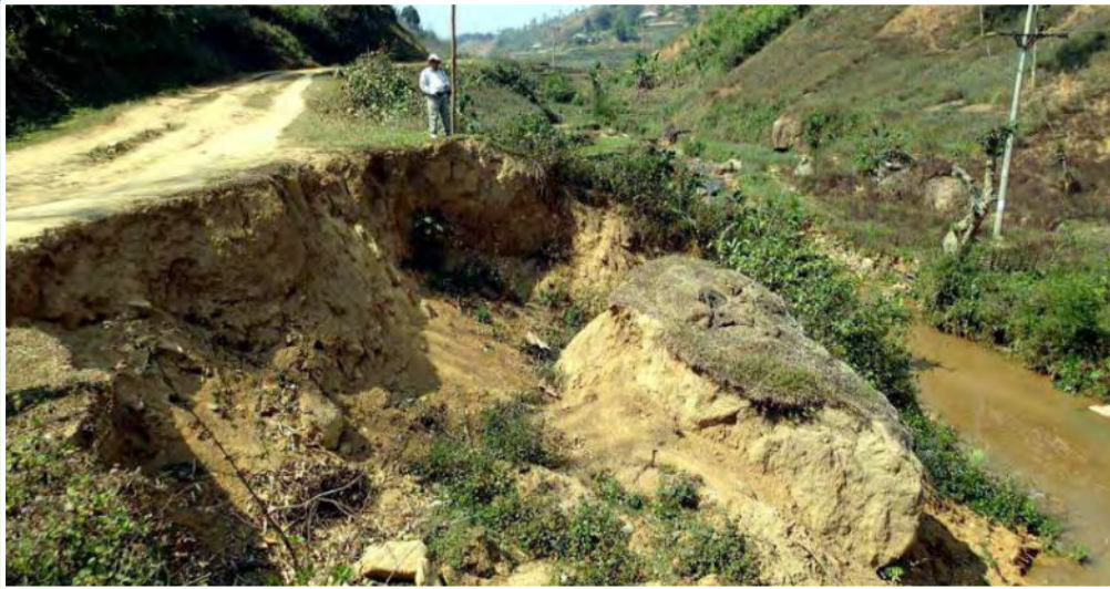
Slope failures
