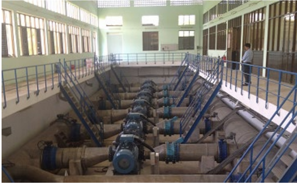
JCM model project on Introduction of High Efficiency Water Pumps at Water Treatment Plant
