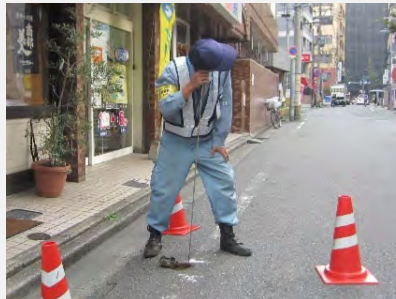
Patrol inspections of underground leakage
