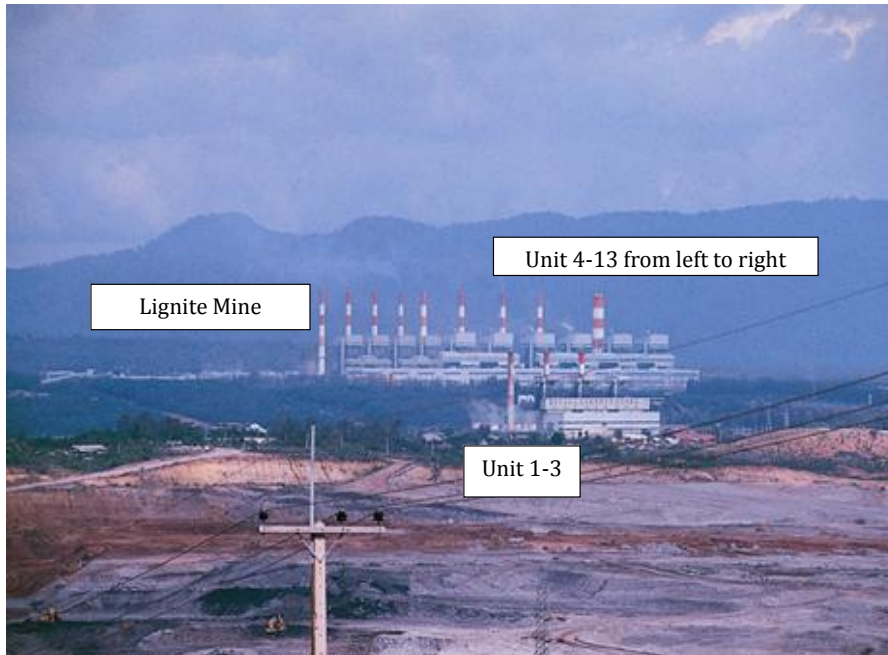
Figure 11. Mae Moh lignite-fired thermal power plant and Mae Moh lignite mine (Source: Pollution Control Department)
