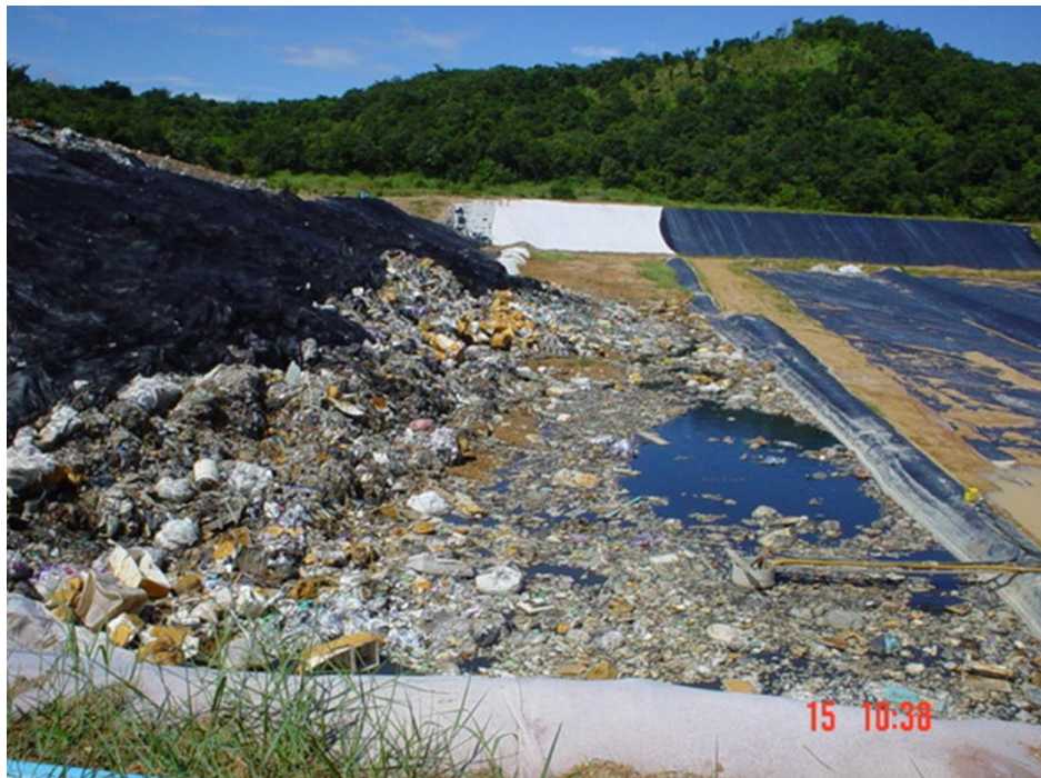
Figure 10. Improper operation of the second sanitary landfill pit after the closure of the first pit (Source: Pollution Control Department)
