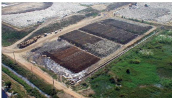
Bio-drying area at MBT facility in Phitsanulok
