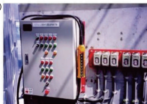
Control panel for remote control
