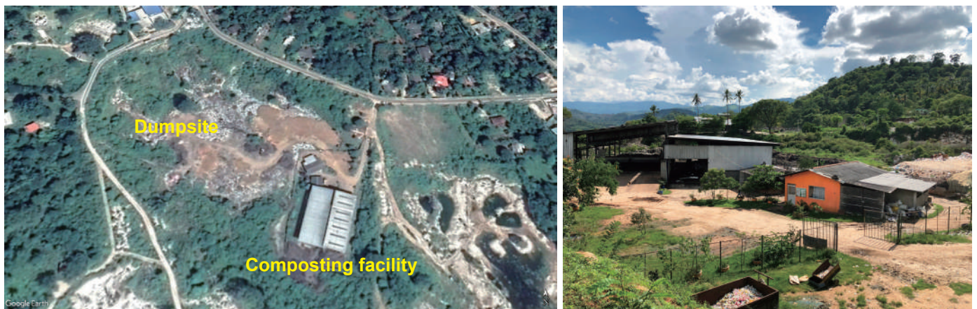
Figure 2-17 Kawashima composting facility at Kundasale PS (Source: author)
