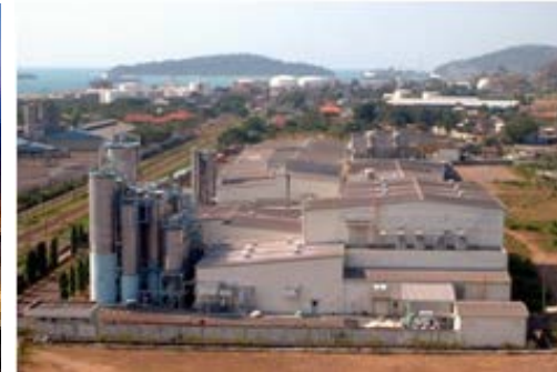
High-efficiency Once-through Boiler System in Film Factory, Indonesia
