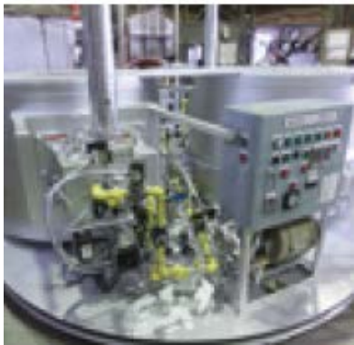
Regenerative Burners to the Aluminum Holding Furnace of the Automotive Components Manufacturer, Indonesia
