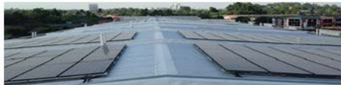
PV power generation system, Malaysia
