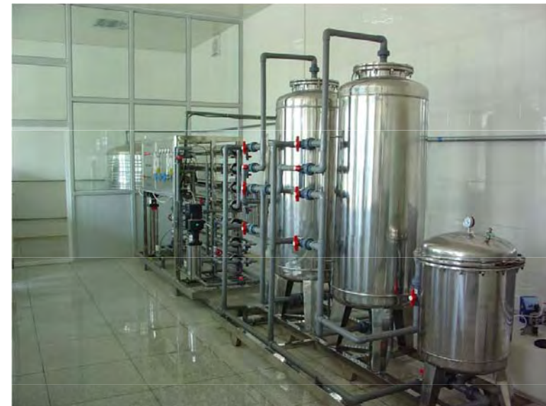
Groundwater treatment plant in Tianjin 5
