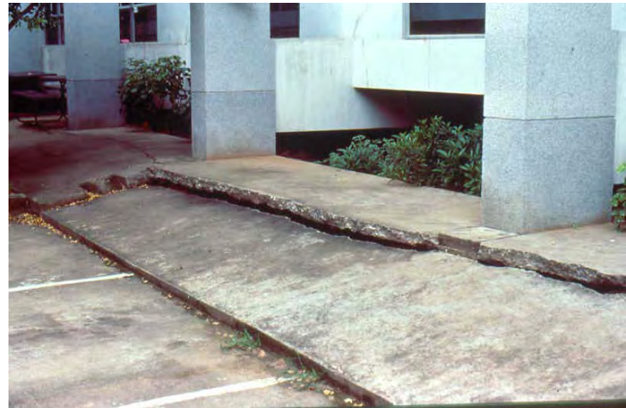
Impact of Land subsidence in Bangkok
