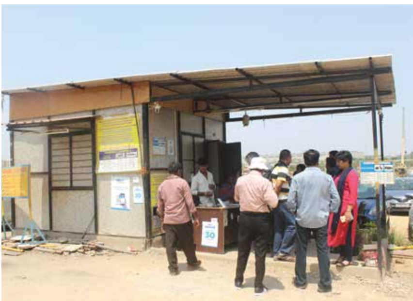
Figure 39: Security staff kiosk made using recycled plastic (left), dust bins made of recycled plastic (right)
