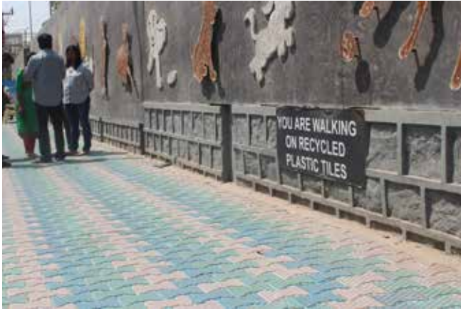
Figure 38: Recycled plastic paver blocks used for making pavements, Dogpark, GHMC
