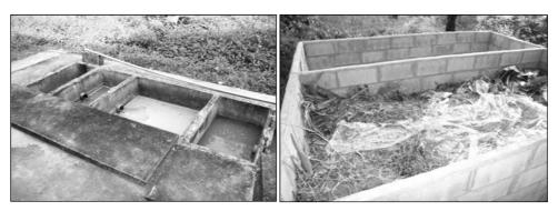
Picture 8: Grease Trap and 'Brew' Pool for organic fertiliser
