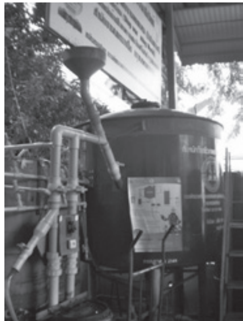
Figure 4.4 A small-scale anaerobic digestion tank
