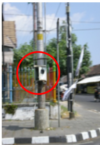
Figure 6.1 kWh Meter in Public Streetlights
