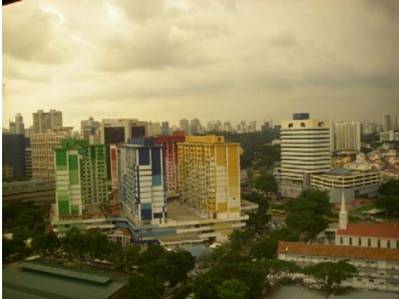
Figure 4.4: Green spaces and green design are critical factors for urban planning in Singapore. The colourful buildings are public housing where more than 80% of Singaporeans reside. (Photo credit R. Kipp, September, 2008)
