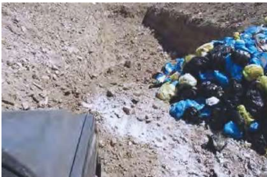
Figure 14 - Burial in special cells in dumping
