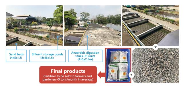
Figure 7. Nonthaburi city faecal sludge treatment plan and fertilizer produced as final product
