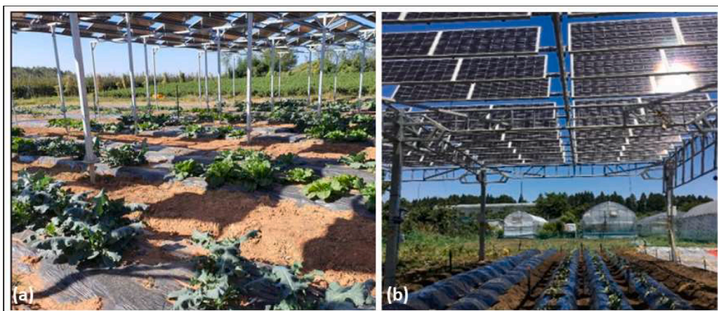
Fig. 1. Tilted solar panels installed on platforms above crops. Photos from Chae et al. (2022) (a) and Yajima et al. (2023) (b).
