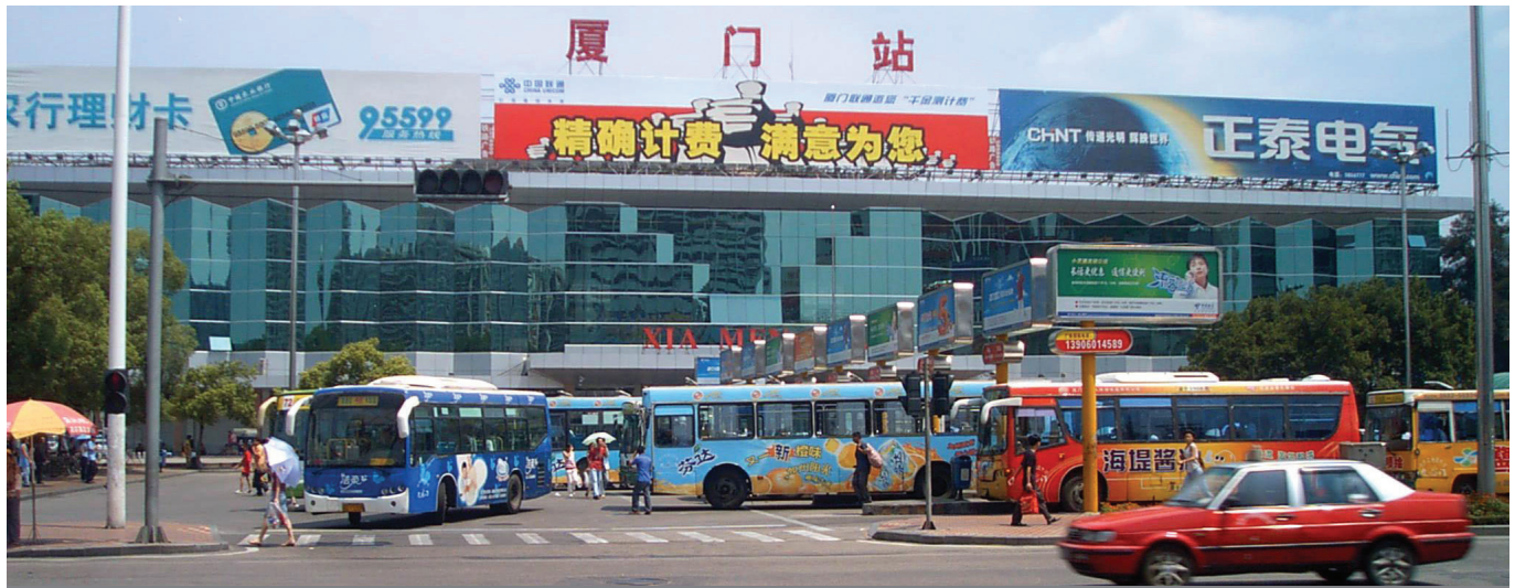
Xiamen Railway Station, Fujian Province, China. Photo by Xmhaoyu / Wikimedia Commons (Licensed under CC BY 3.0).
