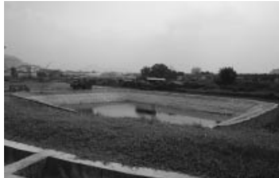
Sanitary landfill underway at a Kuala Lumpur dumpsite (photo : ISIS Malaysia)
