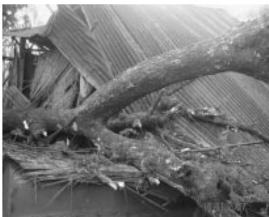
House razed to ground by the cyclone SIDR ©BCAS
