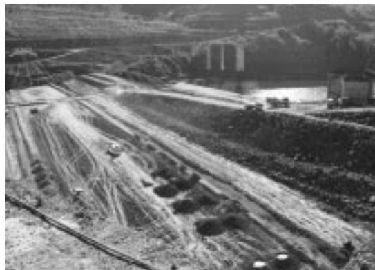
Kun Hydropower Dam Construction Site in the Pegu Yoma Mountain Range
