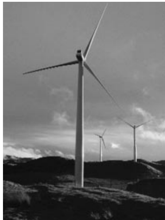
Te Apiti Wind Farm near Palmerston North, North Island Source: Meridian Energy
