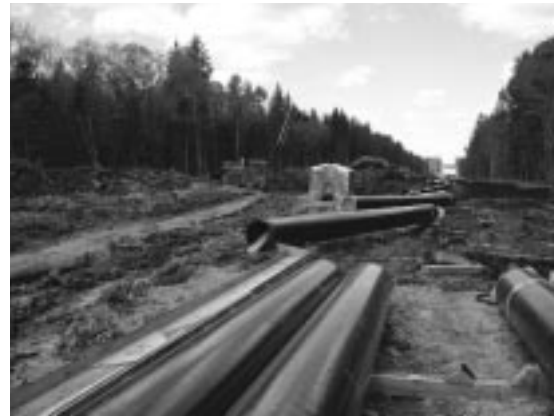
Oil pipeline construction by Sakhalin Energy, violated a set of laws. By D. Lisitzyn
