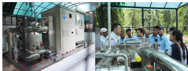
Figure 1. (L) EHP system in dairy plant; (R) onsite training in maintenance and trouble-shooting
