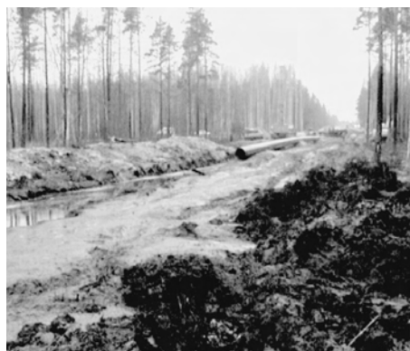
Oil pipeline construction on the Baltic Sea coast area. Copyright©Alexander Sutyagin, project “Monitoring BTS” (Baltic Pipeline System)
