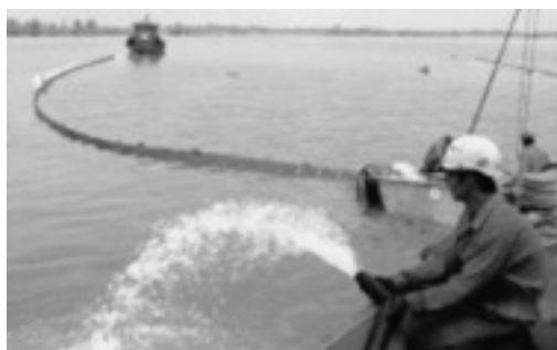
サイゴン川水面の流出油の処理 Trace of the oil-slick on the river surface has been under control.
