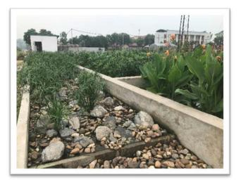
**Figure 2.** A decentralised wastewater system constructed in Hanoi, using nature-based technologies
