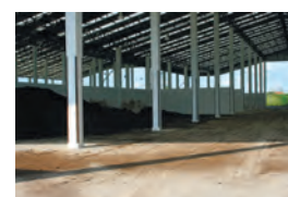
An underutilised building in On Nut Waste Transport Station that could be used as a centralised composting centre
