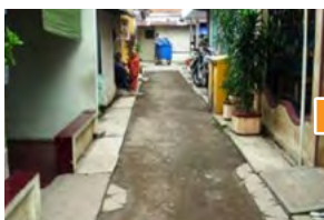
A street before implementation of the project.
