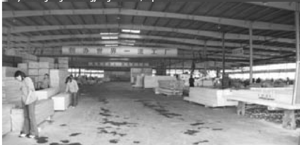
Figure 9 A large wood product manufacturing enterprise located in the Chinese border city of Dongning - Heilongjiang Province, Sept. 2006
